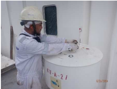
10) Shutting off ventilations
