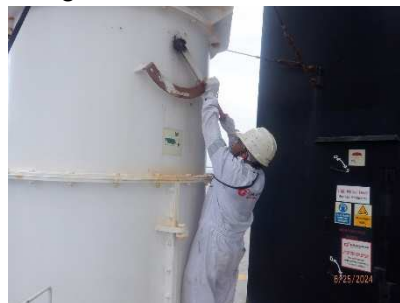
8) Shutting off ventilation
